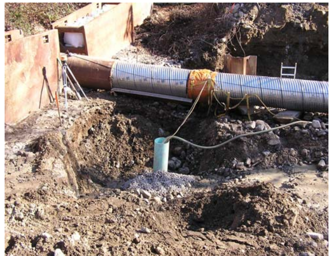
Stream Bypass Piping and Dewatering Pit
