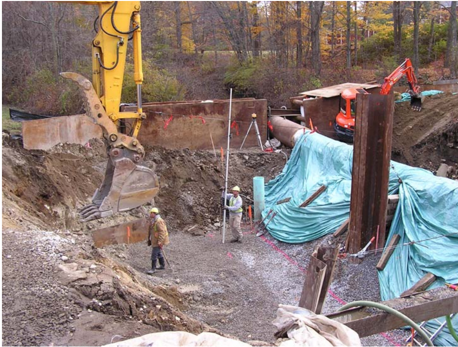
Excavated Area Being Prepared for New Footing
