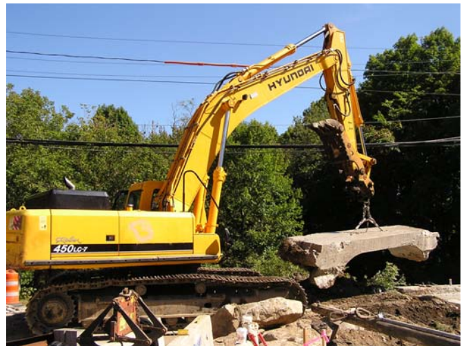
Demolition and Removal of Existing Bridge Decking and Superstructure
