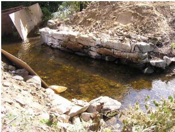
Old Stone Bridge Abutment Prior to Removal
