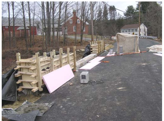
bridge rail concrete work prior to removing formwork
