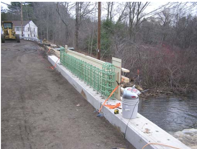
bridge rail reinforcing steel
