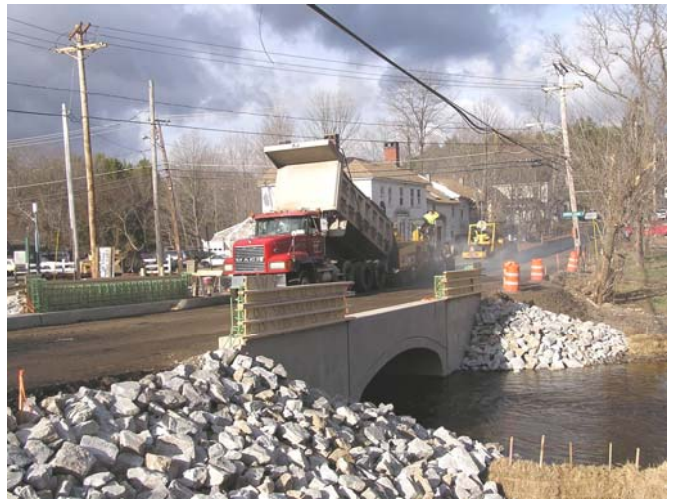
binder course paving of road
